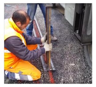
Fig. 8: Insertion of the post type IPE 80 with welded Fig. 9: Tool for the post hammering screwed on the plate.
