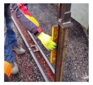
Fig. 10: Check through the spirit level
