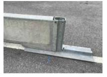
Place a start/end element on one side of the pillar and, with the aid of a crane, lift an element into position on the other side of the pillar.
