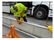
Once the element is standing on the ground, undo one of the lifting clamps. The crane will ensure the lifting chain in the remaining lifting clamp is held taut.
